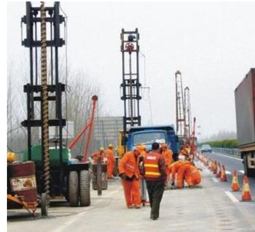
Vibro-squeezing sand pile reinforcement method
