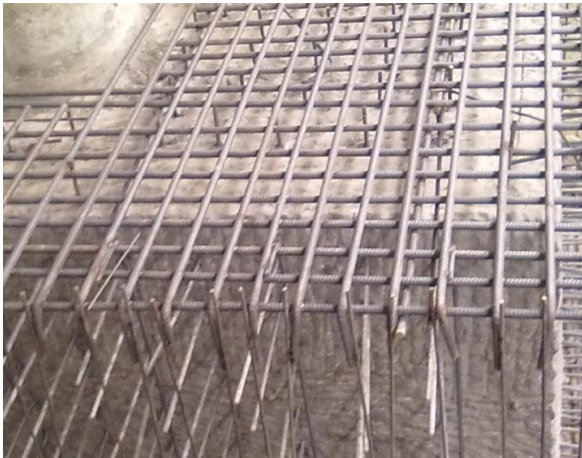
Reinforced method of bending strength of pile caps
