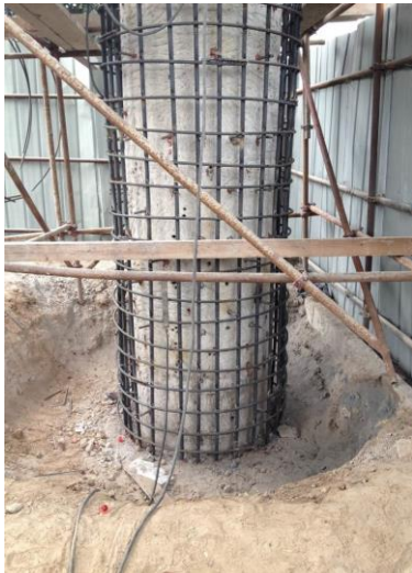
1. Enlarging section method
