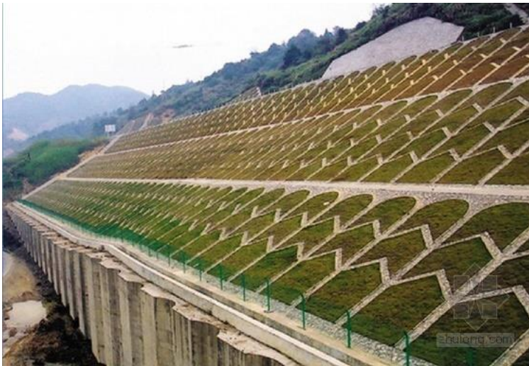
Slope Protection of retaining wall
