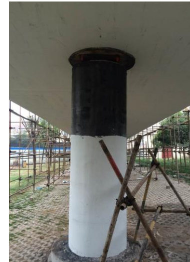
3. Sticking fiber composite material method
