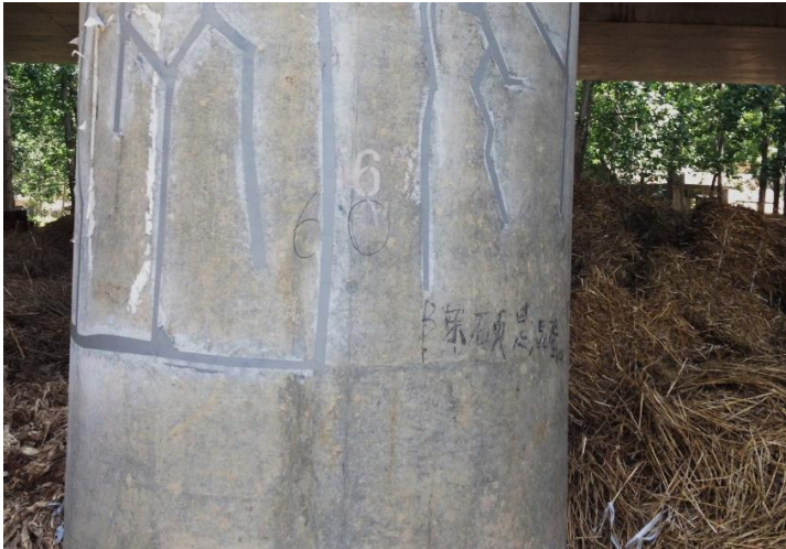
Pier and pillar defects fixing
