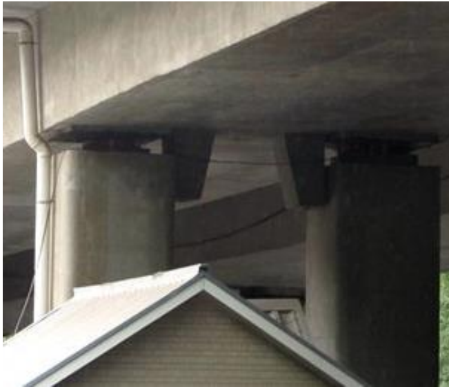
The Seismic Block of continuous beam
