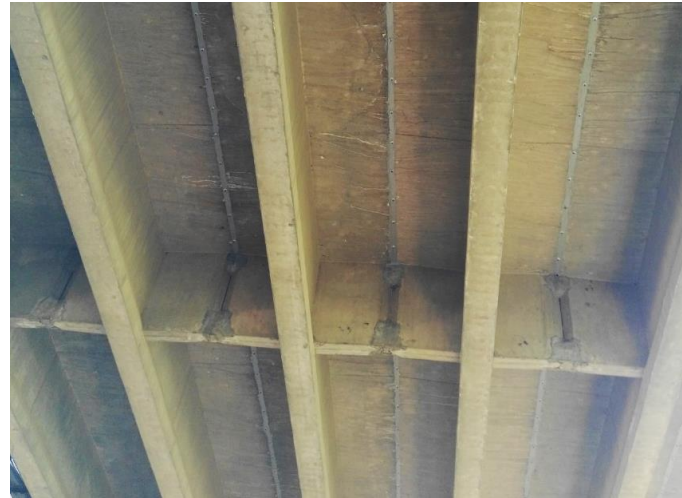
Hinge joints grouting sealing
