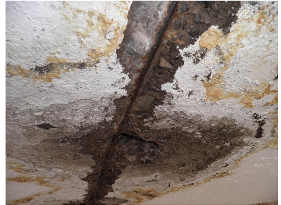
Beam and plate joint corrosion
