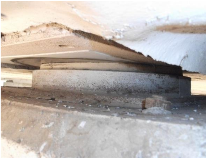
Bearing slip and offset
