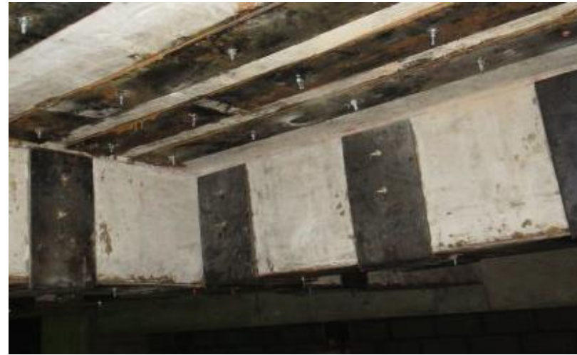
Externally bonded steel plates
