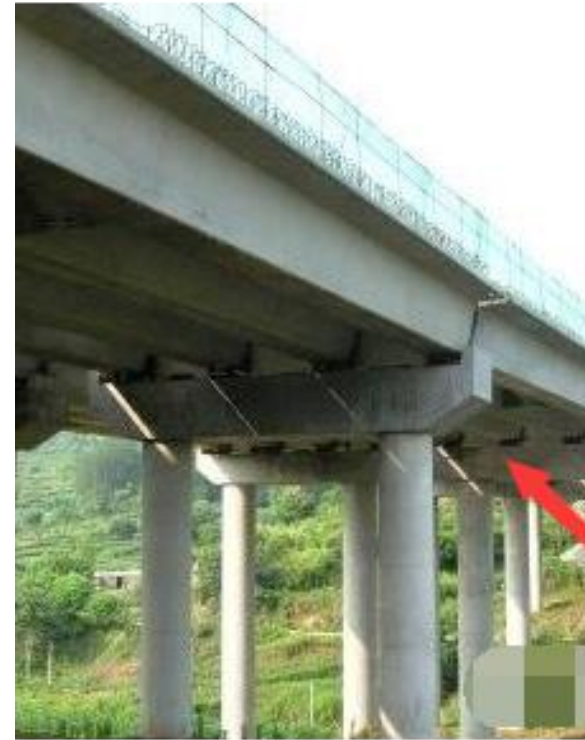
The Seismic Block of bent cap
