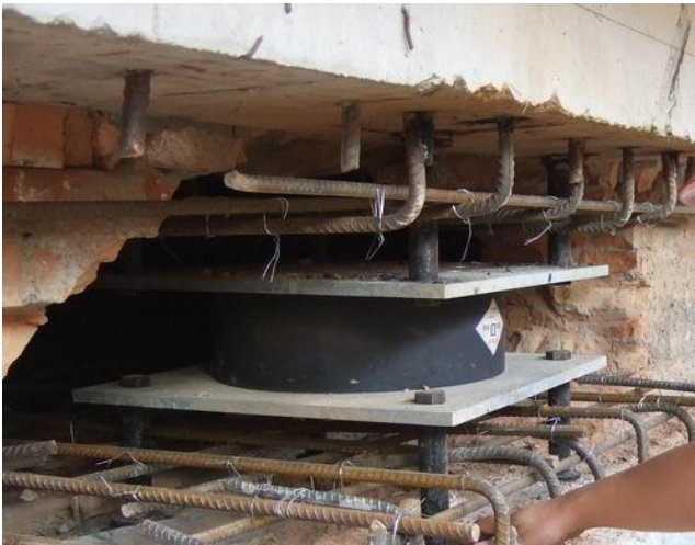
Replacement of isolation bearings
