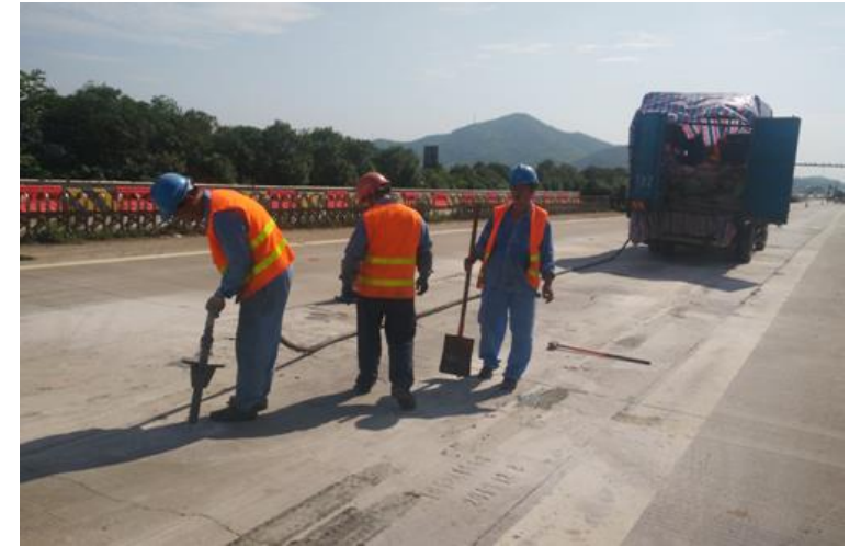
Subgrade compaction grouting
