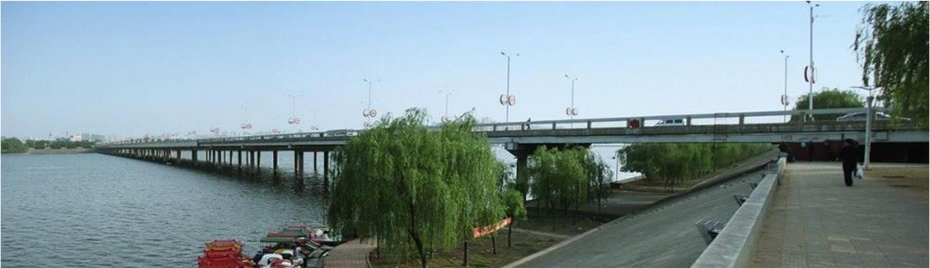
The Luoyang Peony Bridge is 1369.65m long with 34 width. **The earthquake fortification is lever B, and seismic fortification intensity grade is 8.** The peony bridge is composed of main bridge and approach. The main bridge across the Luohe River, and the approach is viaduct connecting Jiefang Road. **The reinforcement for the approach is the main part of this work.**
