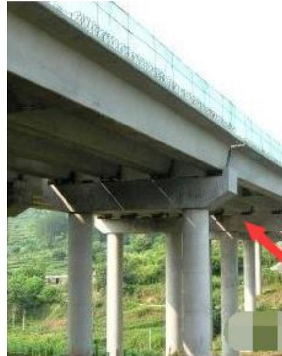
The Seismic Block of bent cap
