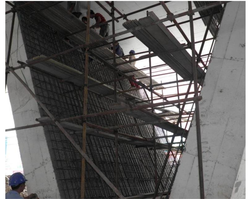
Enlarge the section of V type pier
