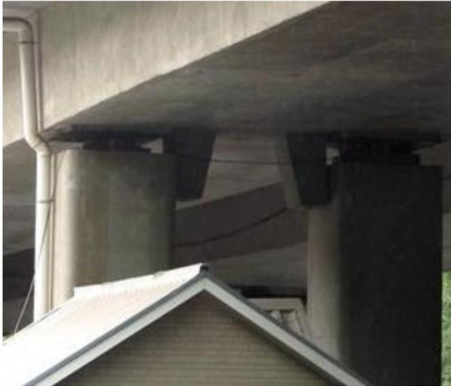
The Seismic Block of continuous beam
