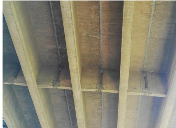
Hinge joints grouting sealing
