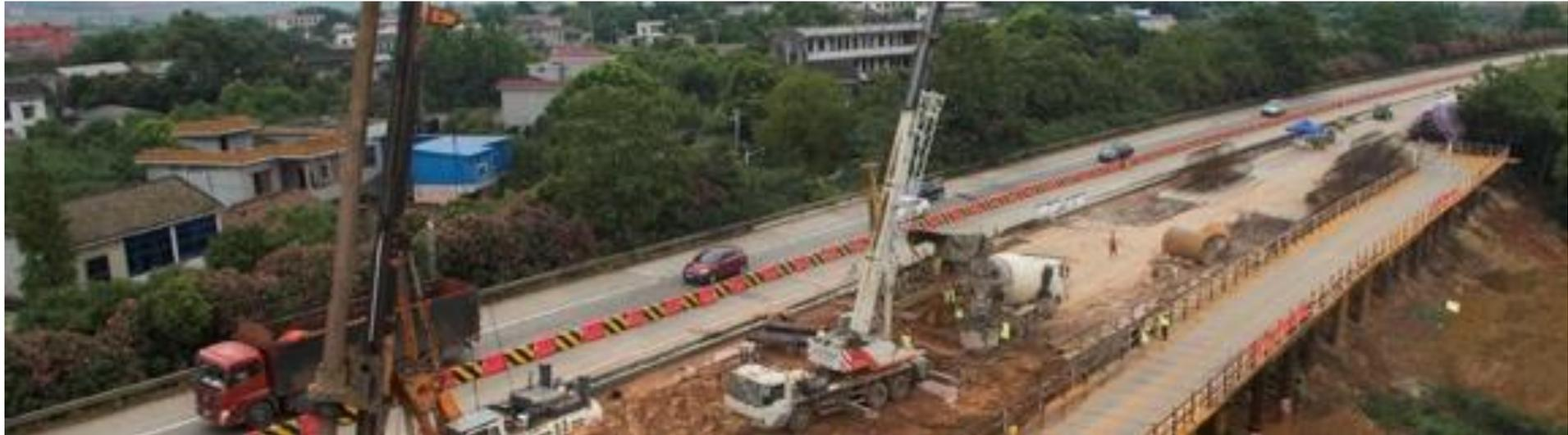
G60 Highway is a main part of National Highway Project, its section in Hunan province is called Xiangtan-Shaoyang Highway (also Tan-Shao Highway), which links Xiangtan, Loudi and Shaoyang with a total length of 220.1 km. The Tan-Shao highway is **designed with four lanes, Seismic fortification Level B, Seismic fortification Intensity Grade 7**. It is **built with concrete surface, and the other 146.620km is bituminous concrete**.
