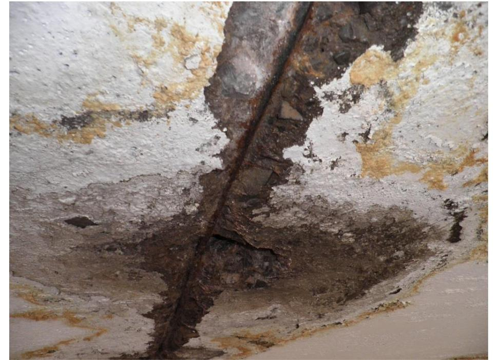
Beam and plate joint corrosion
