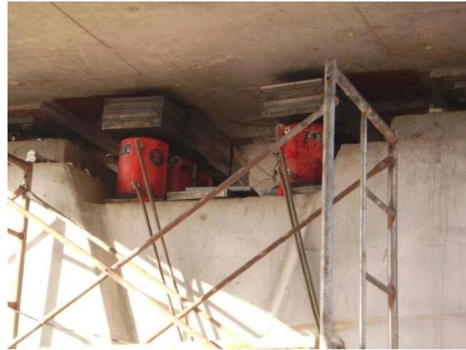
Replacement lift of isolated bearings
