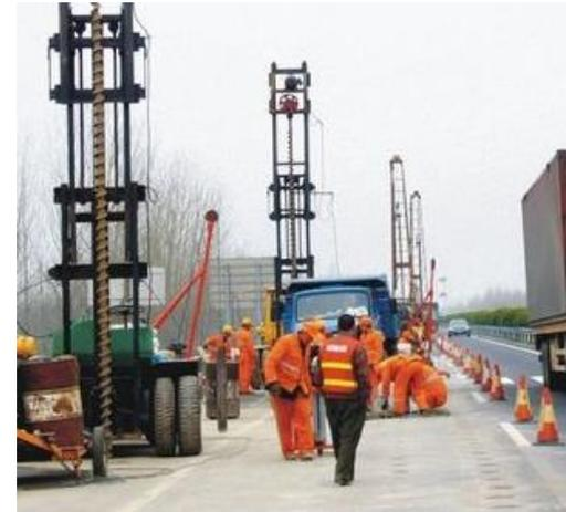
Vibro-squeezing sand pile reinforcement method
