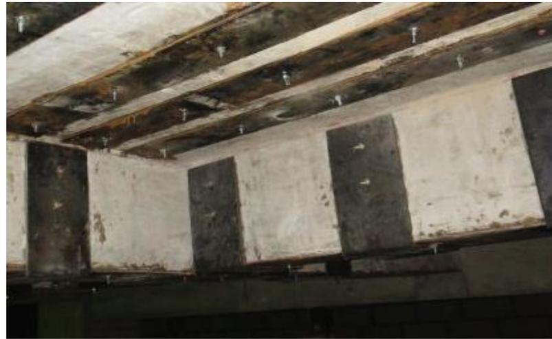
Externally bonded steel plates
