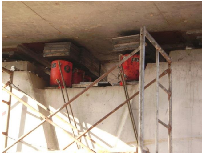
Replacement lift of isolated bearings
