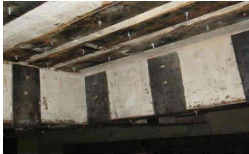
Externally bonded steel plates
