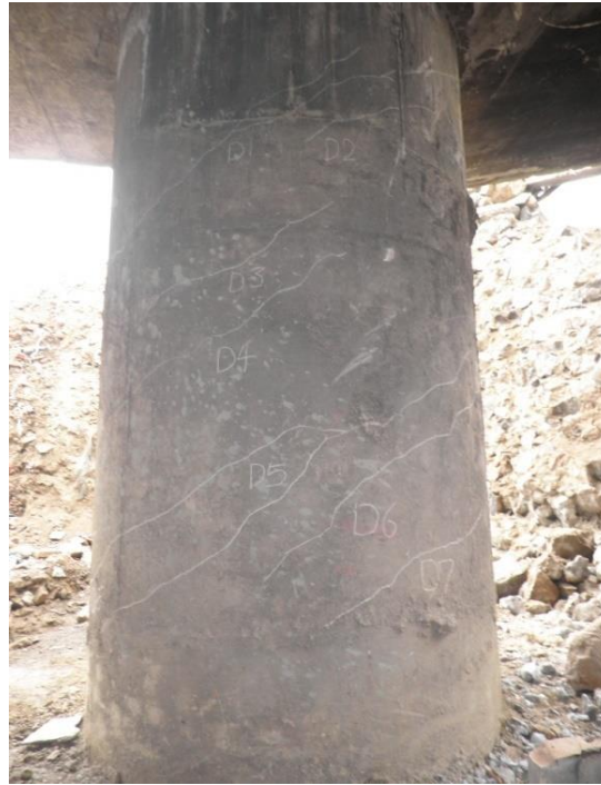
Transverse crack
