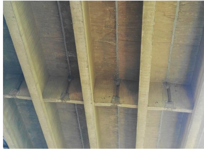
Hinge joints grouting sealing
