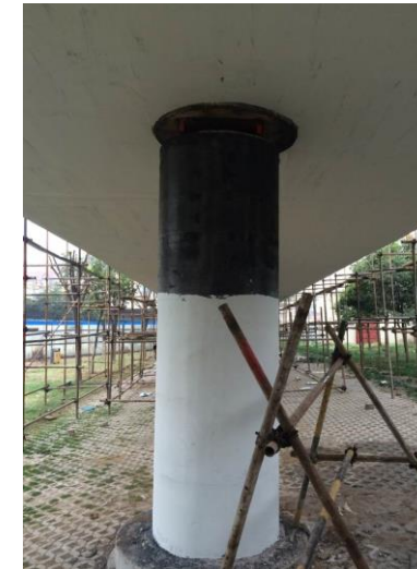
3. Sticking fiber composite material method
