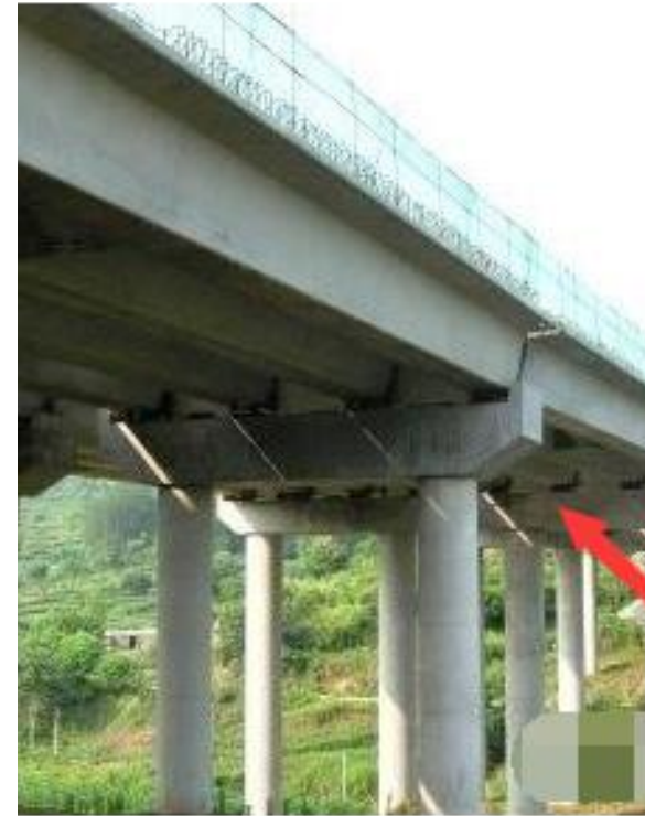
The Seismic Block of bent cap
