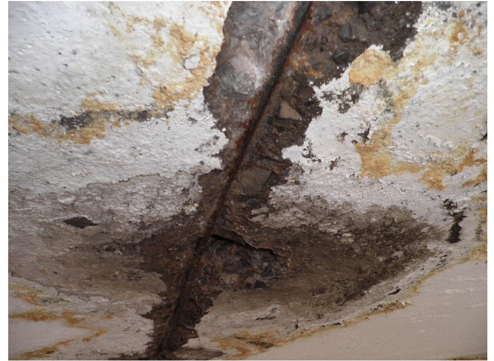
Beam and plate joint corrosion
