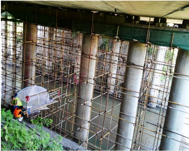
Bearings replacing
