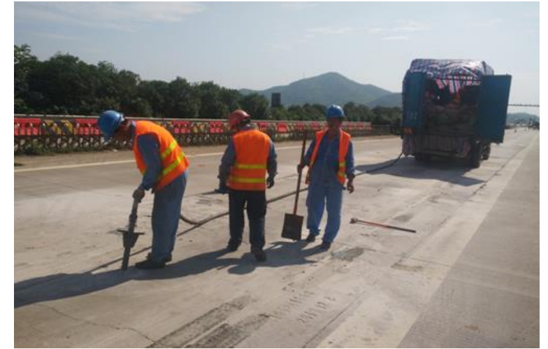
Subgrade compaction grouting
