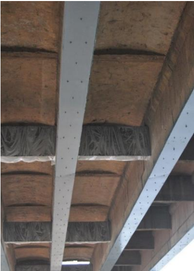
Stick Steel Strengthening Method
