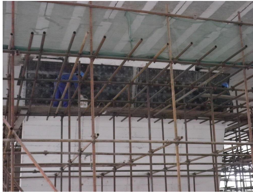
Bond steel plate at the top of all middle piers
