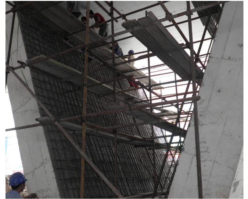
Enlarge the section of V type pier
