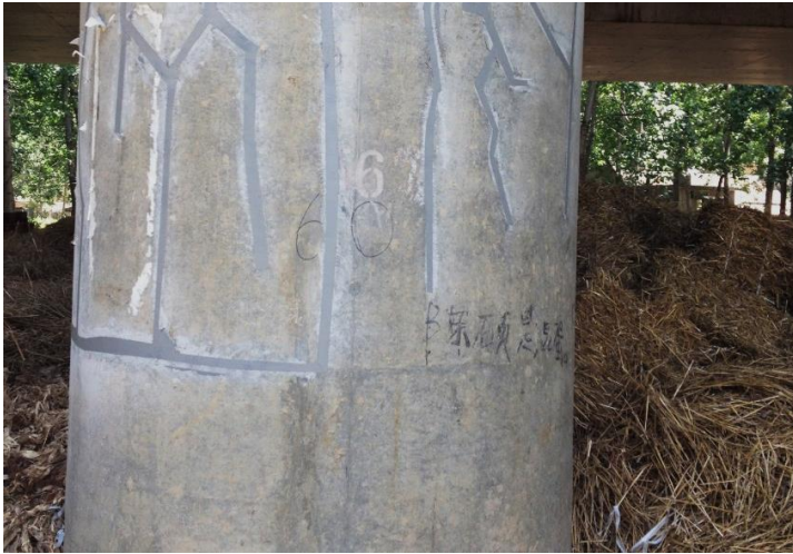
Pier and pillar defects fixing
